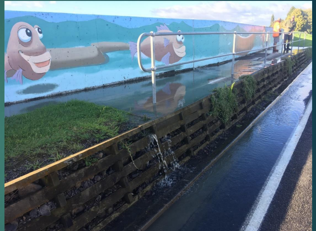
College Road Floodwall Source: Bay of Plenty Regional Council, 2017
