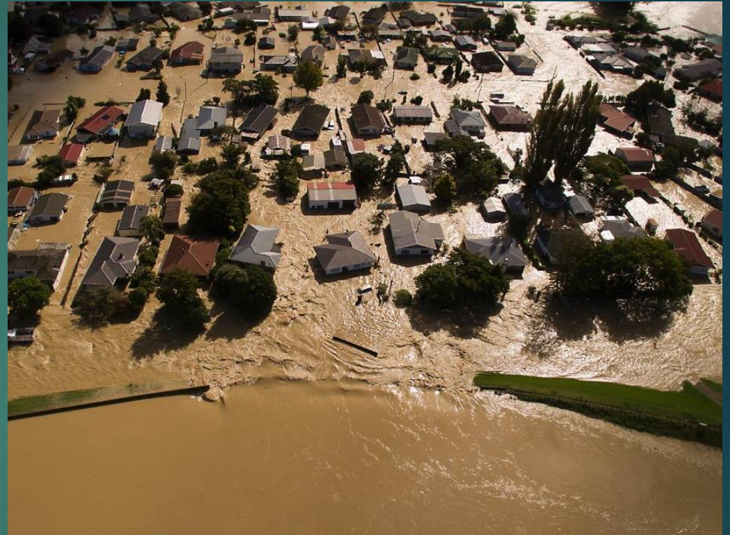
Breached College Road Floodwall Source: Chris McKeen, Fairfax New Zealand, 2017
