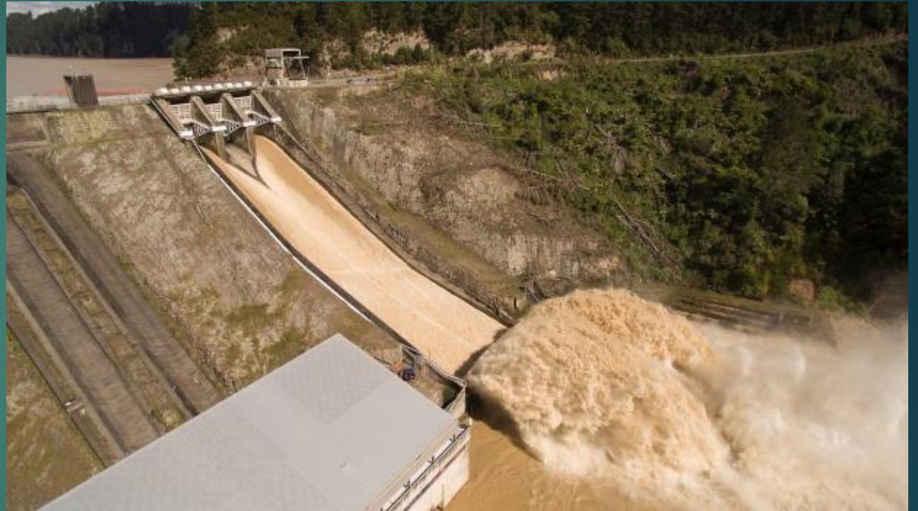
Matahina Dam spillway during 2017 event Source: Chris McKeen, Fairfax New Zealand, 2017
