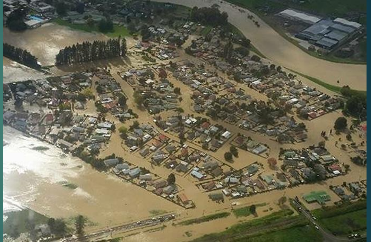
Breached College Road Floodwall Source: Malcolm Growden, 2017
