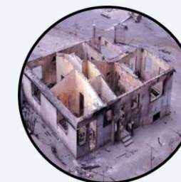
Fire damage from low momentum PDC, 1997 eruption of Soufrière Hills, Montserrat. Credit Baxter, P., (2005), Bul. Volc.
