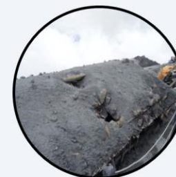
Roof, with wind protection boulders, covered in ash <500m from 2014 Mt Ontake eruption, Japan. Credit Kae Tsunematsu.
