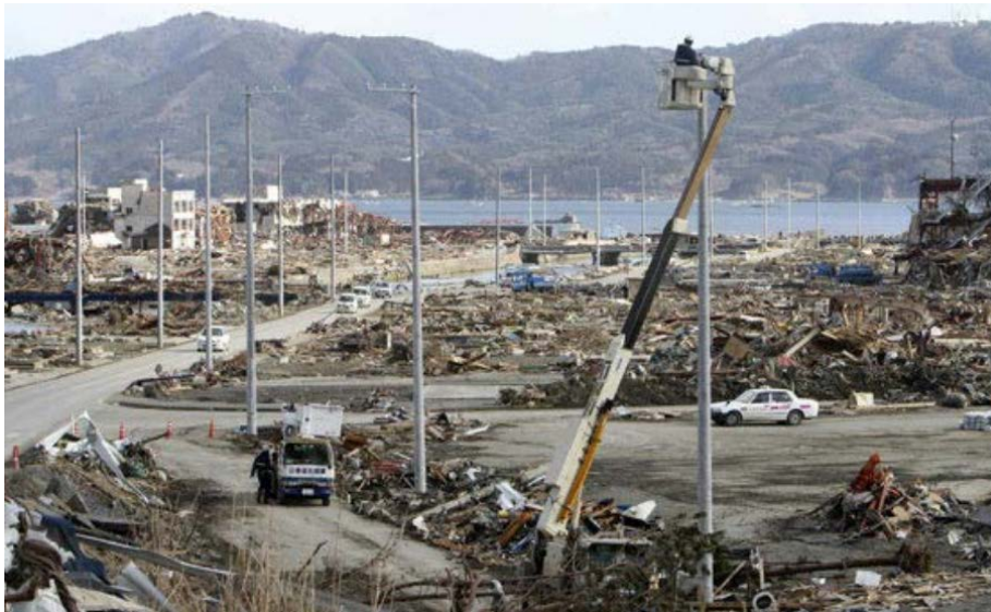
Utility poles being reinstated following the 2011 Japan Tsunami
