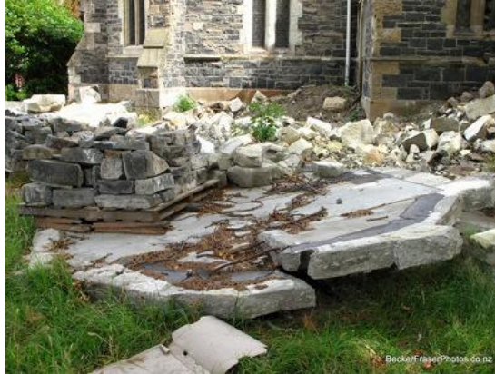
[2] Scattered masonry that has fallen from St John the Baptist Church in Latimer Square
