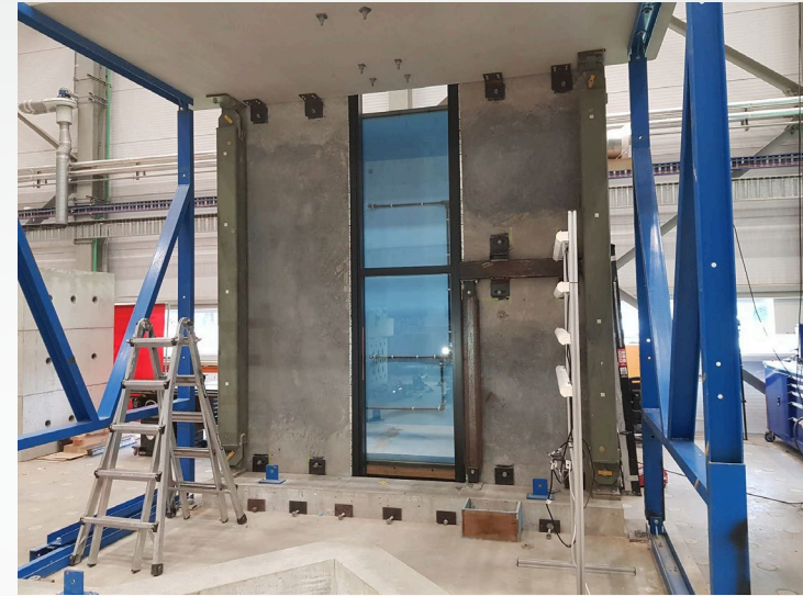
Figure 8: Photo of the current progress of the test setup, with the precast panels and the seismic glazing system installed.
