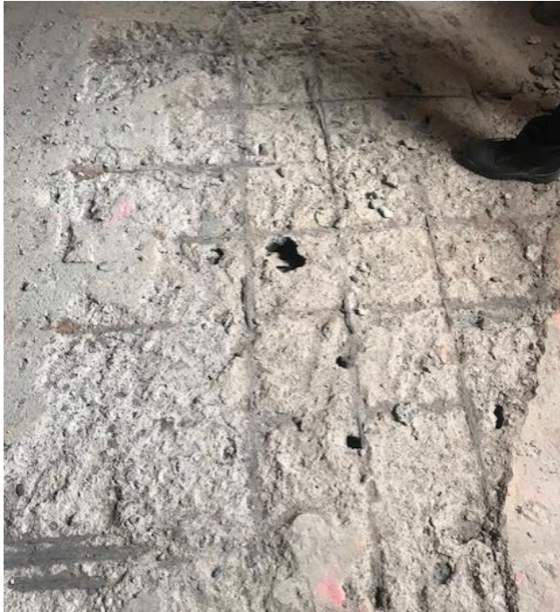
(a) The floor before FRP installation
