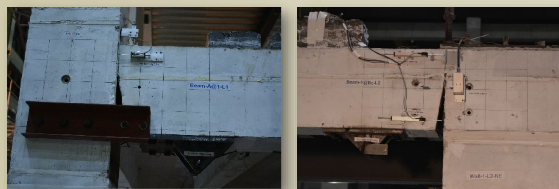
Figure 4 Final condition of slotted beam joints
