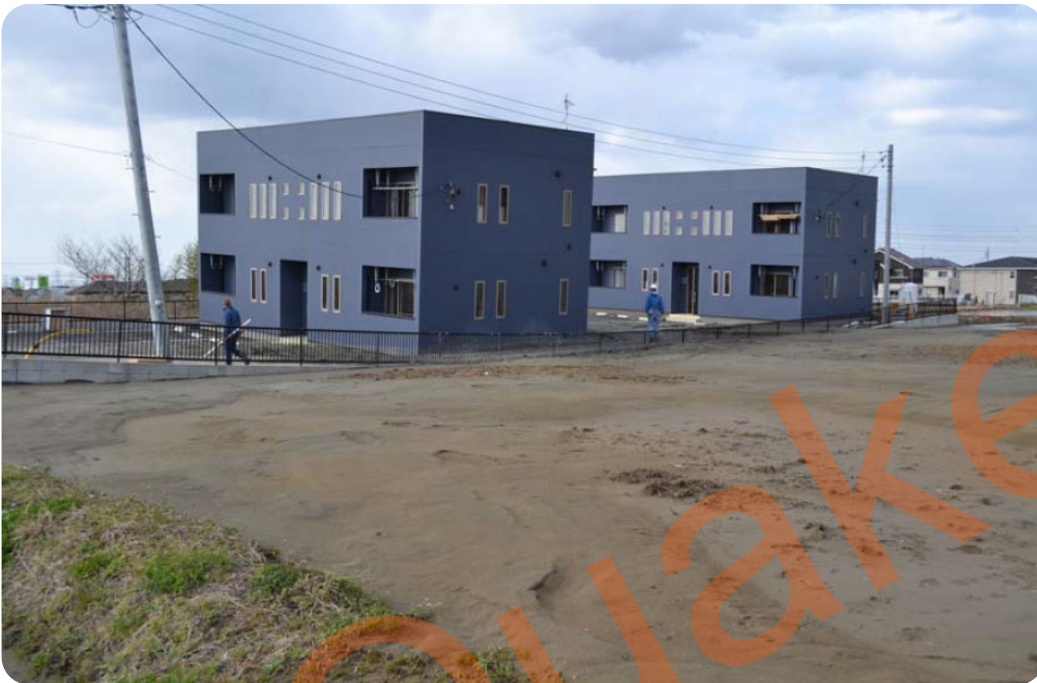
Settlement of structures during 2011 Tohoku earthquake, Japan (Ashford et al., 2017)
