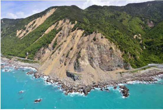
Debris and rock avalanches in greywacke along State Highway 1, triggered by the Kaikoura EQ (Photo: D. Townsend)
