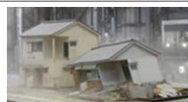
Two-story Wooden House
