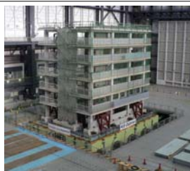
Six-story RC Frame
