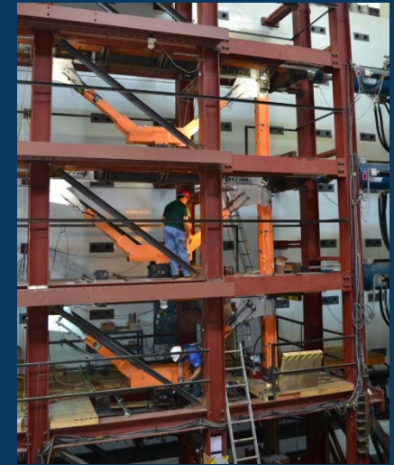
Experimental substructure (DBF)
