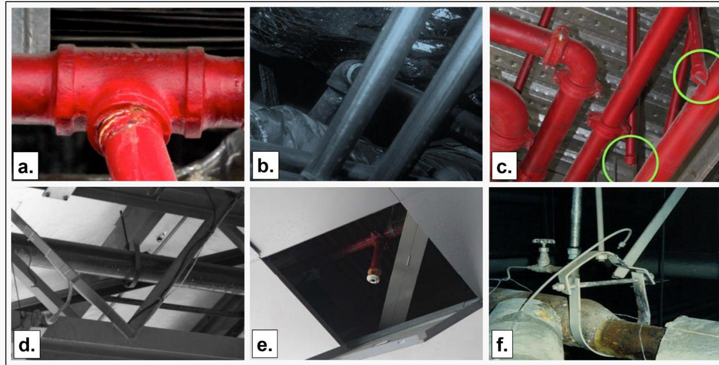
(a) Fractured Tee Joint; (b) Fractured Elbow Joint; (c) Braces Sheared Off; (d) Failure of Hanger; (e) Sprinkler Head Sheared Off; (f) Failure of Brace (Baker et al. 2012)(Miranda et al. 2010)(Taghavi and Miranda 2003)(Tian 2013)
