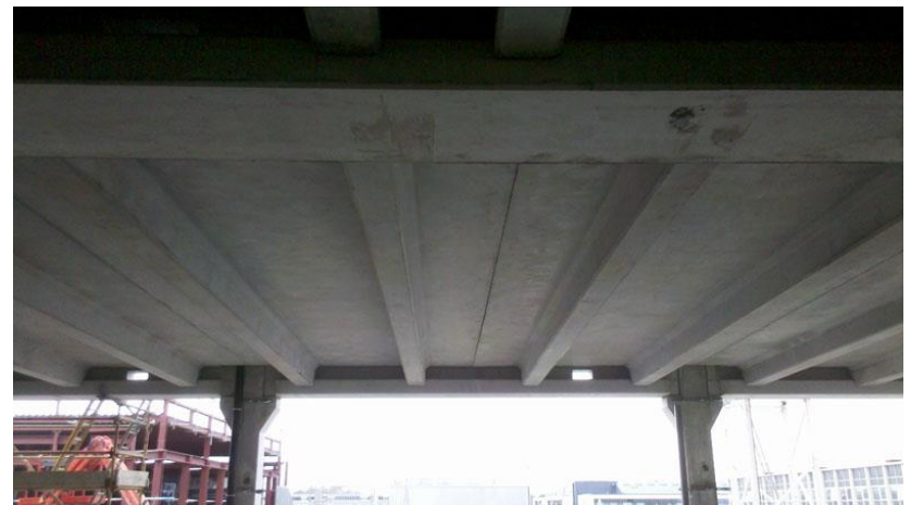
500 Double Tee Typical Section
