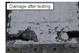
Damage after testing
