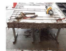
Removal of existing reinforcement
