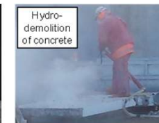
Hydro-demolition of concrete
