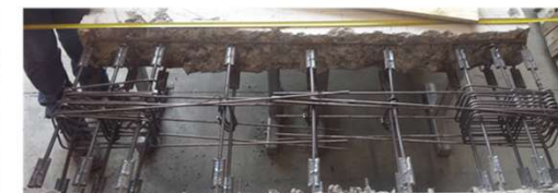
Reinstatement of new reinforcement
