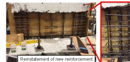
Reinstatement of new reinforcement
