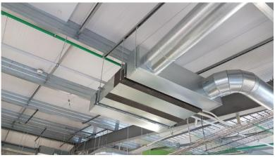
2. Elements that are unable to withstand building deformations
