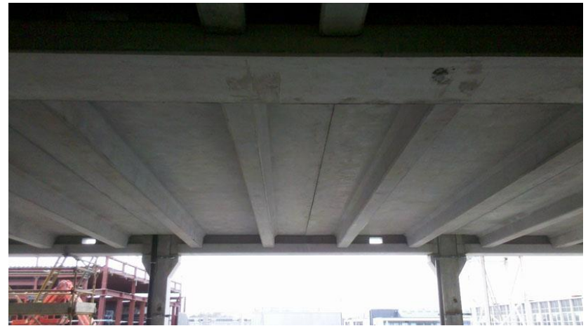
500 Double Tee Typical Section
