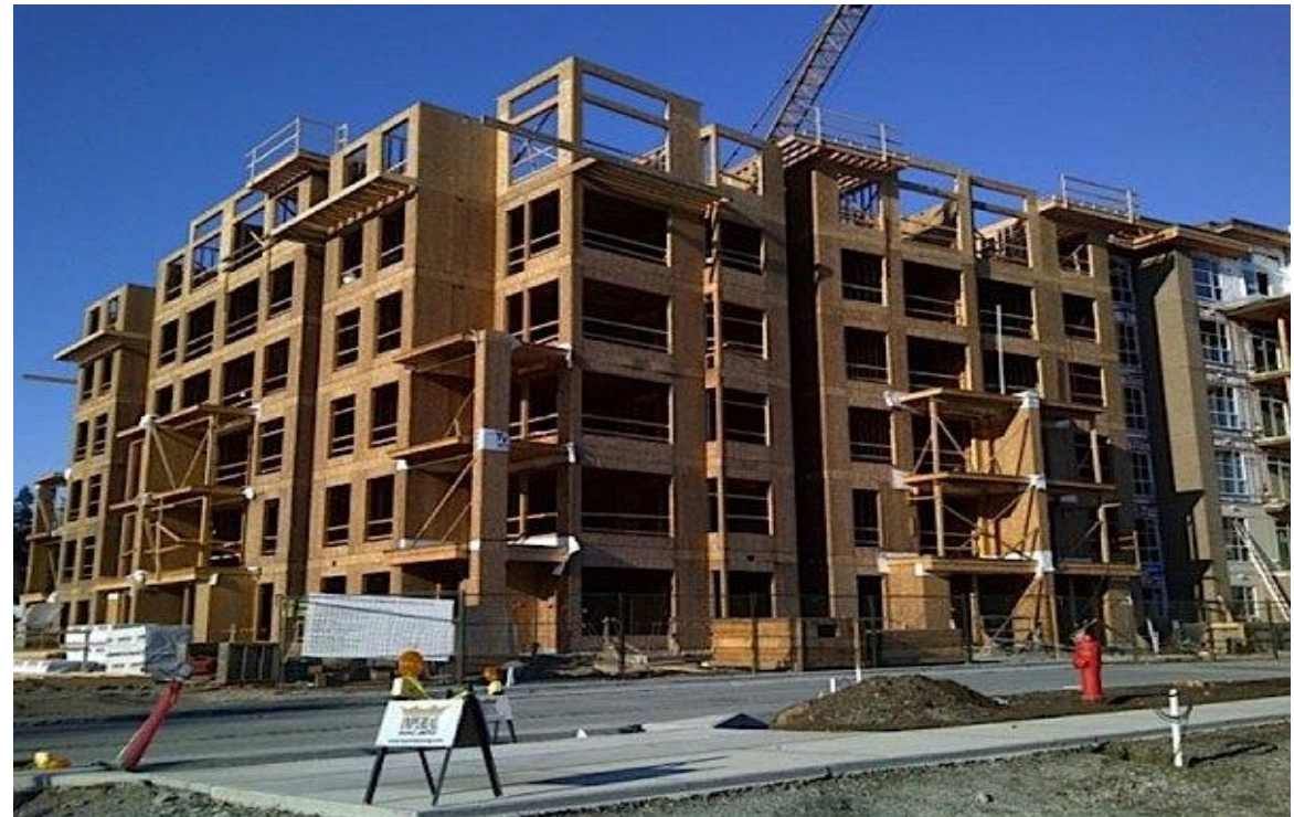
Six Storey Light Timber Frame Construction (On-Site, 2015)
