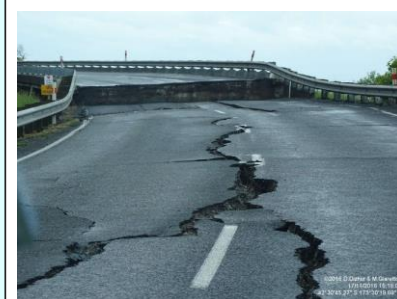
Oaro bridge approach failure and pavement cracking. Photo credit: Dizhur & Giaretton.
