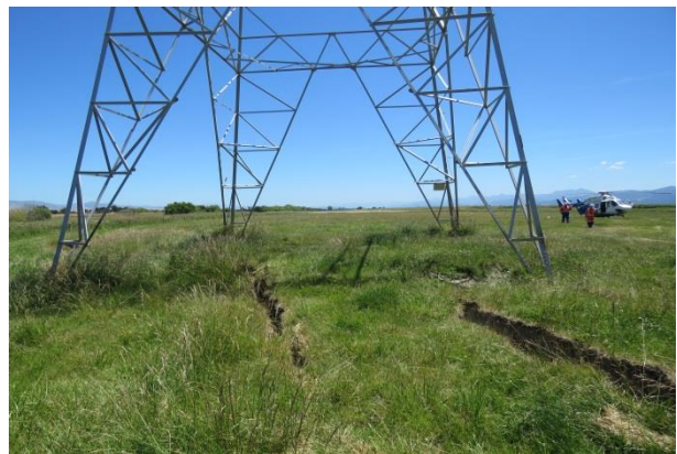
Figure 7: Ground crack between legs of the HVDC tower.
