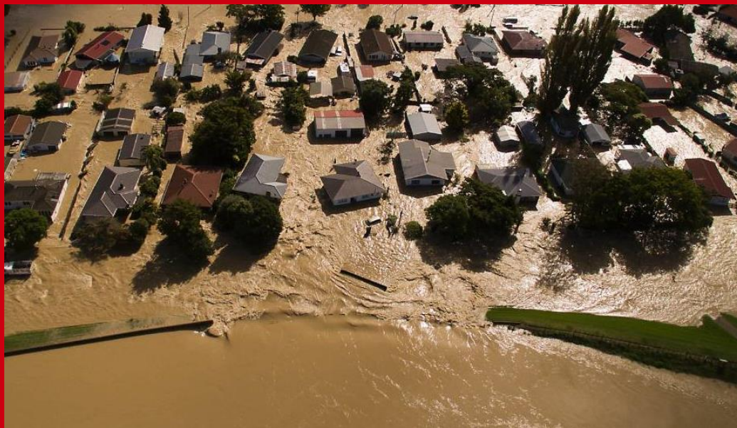
Breached Floodwall in Edgecumbe (Chris McKeen, Fairfax New Zealand, 2017)
