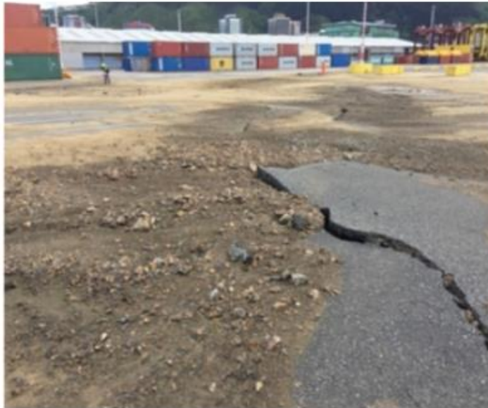
Gravelly soil liquefaction at Centerport, Wellington
