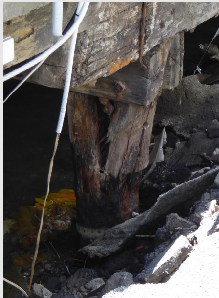
Damage to Thorndon and King's wharf piles and deck (severe)
