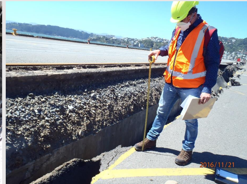
Damage to Thorndon and King's wharf piles and deck (severe)
