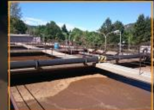
Biological reactors at the municipal wastewater treatment plant at San Martín de los Andes, Argentina, continued to function without problems despite receiving 2 cm of ashfall from the 2015 eruption of Calbuco volcano, 345 km away in Chile. This was partly because the town's storm drains and sewers are well separated, so very little ash entered the plant in raw wastewater. Photo credit: Daniel Blake
