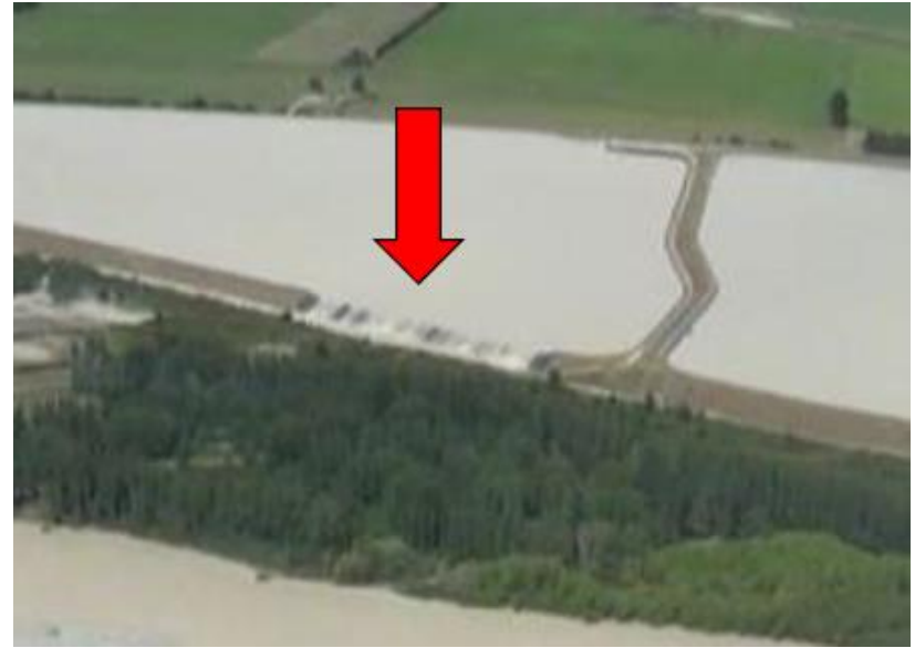
Discharge through pond weir
